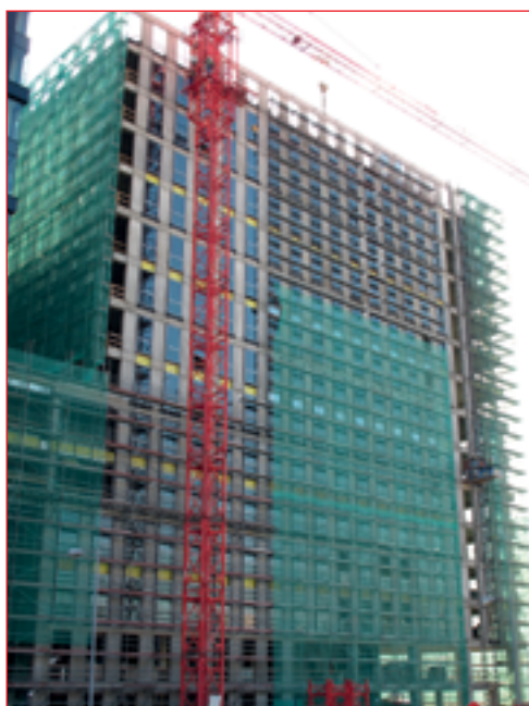
Budowa Quattro Business Park - Kraków
