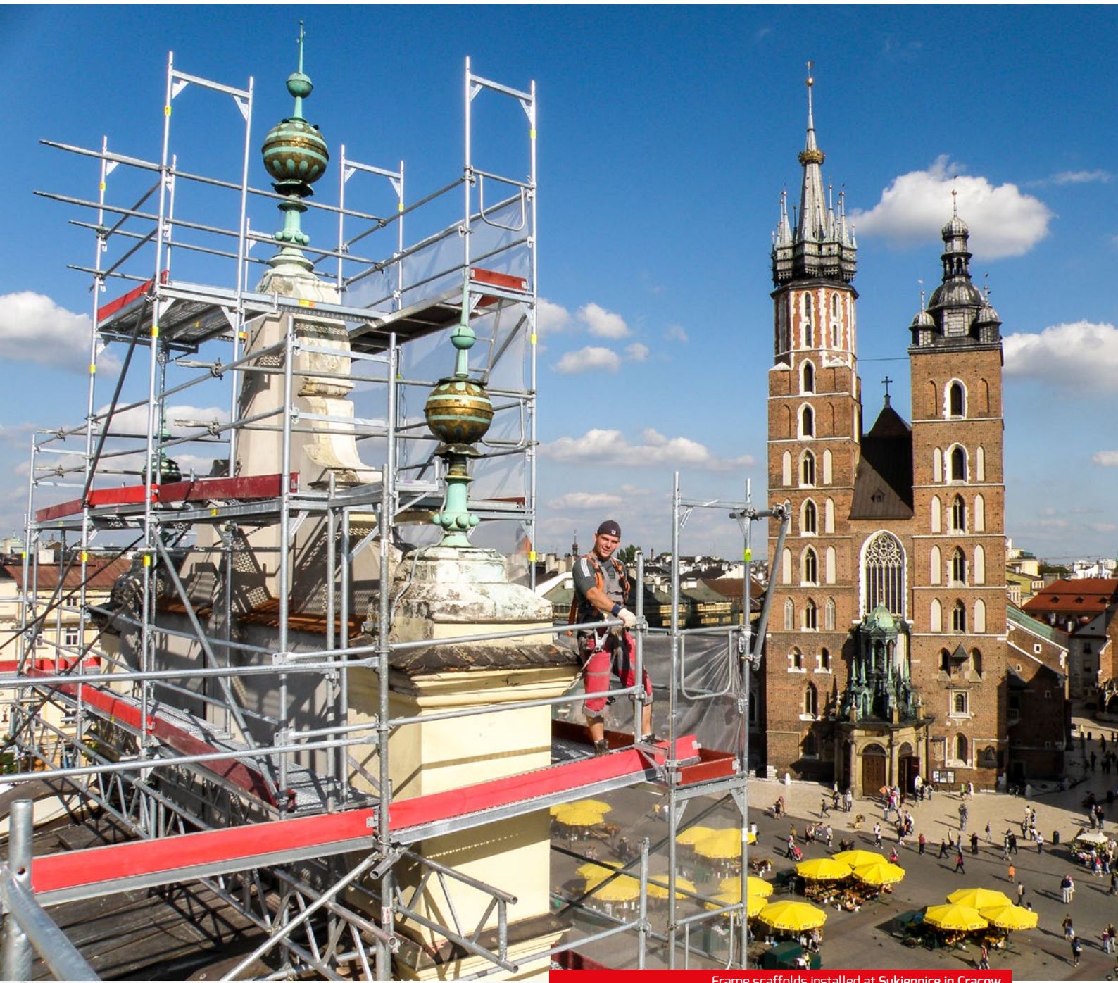
Frame scaffolds installed at Sukiennice in Cracow
