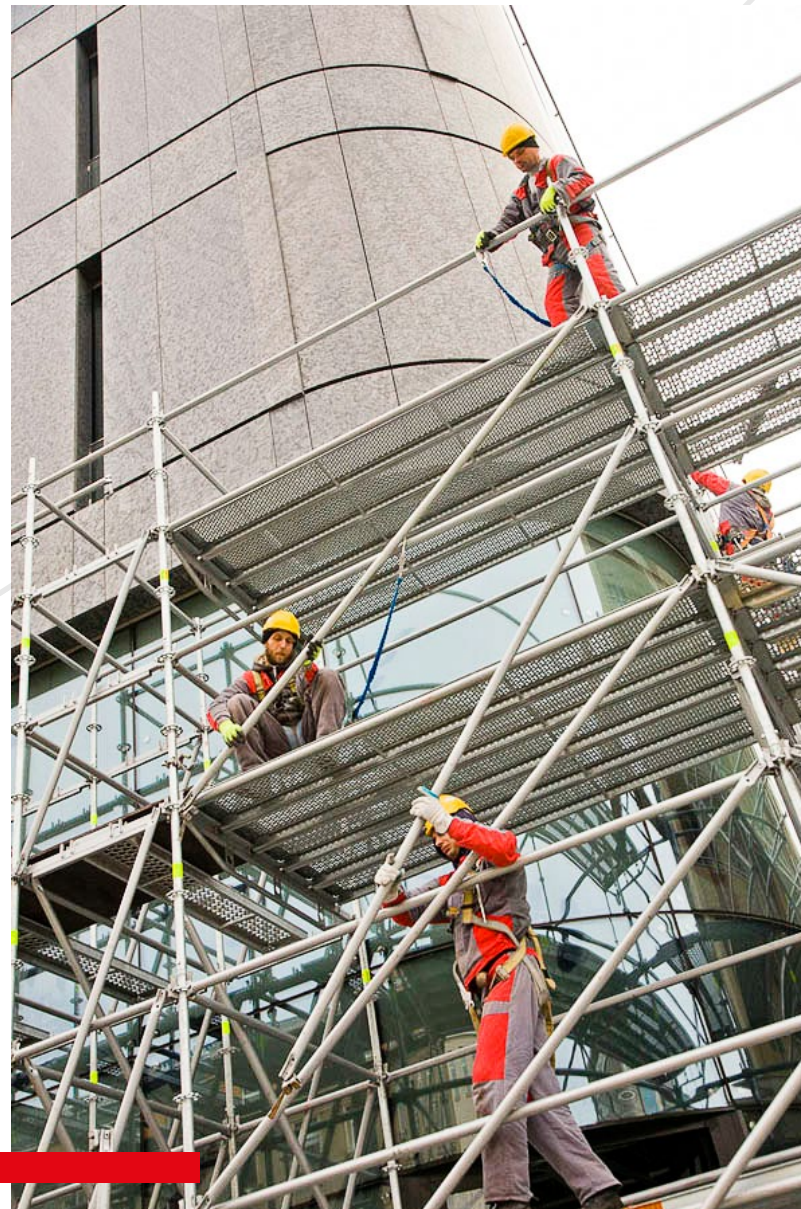
Professional ALTRAD Mostostal Installers Installation
