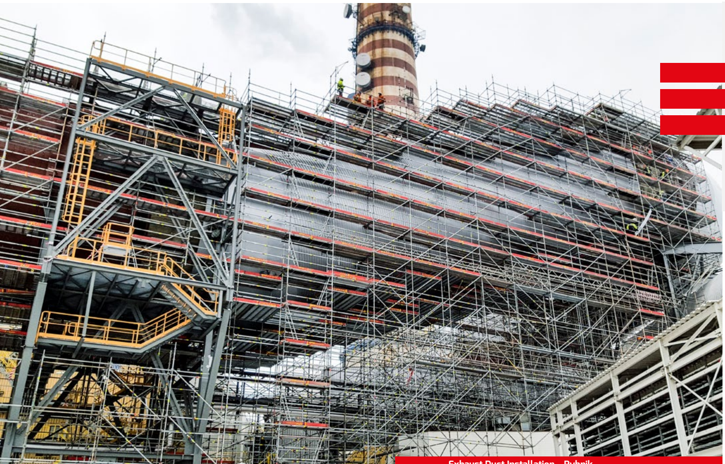
Exhaust Duct Installation – Rybnik
