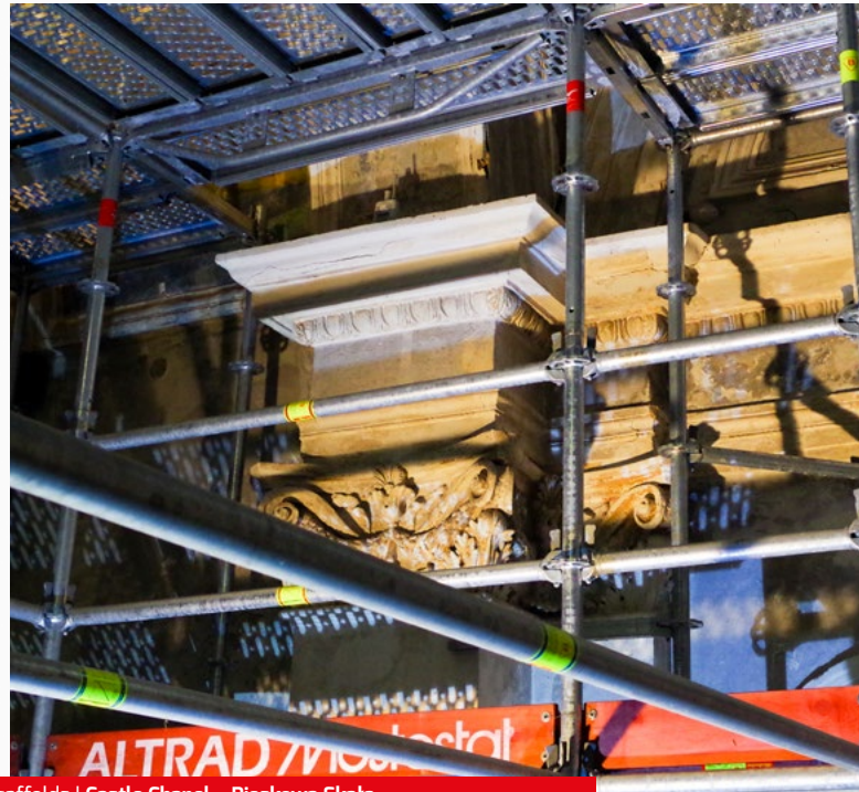
ROTAX Plus Modular Scaffolds | Castle Chapel – Pieskowa Skala
