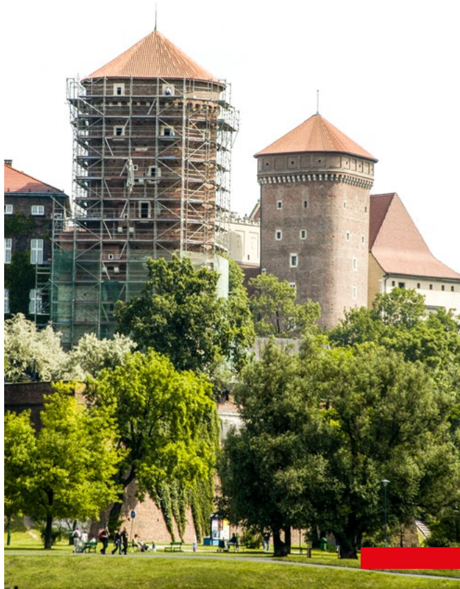
Wawel Tower - Cracow
