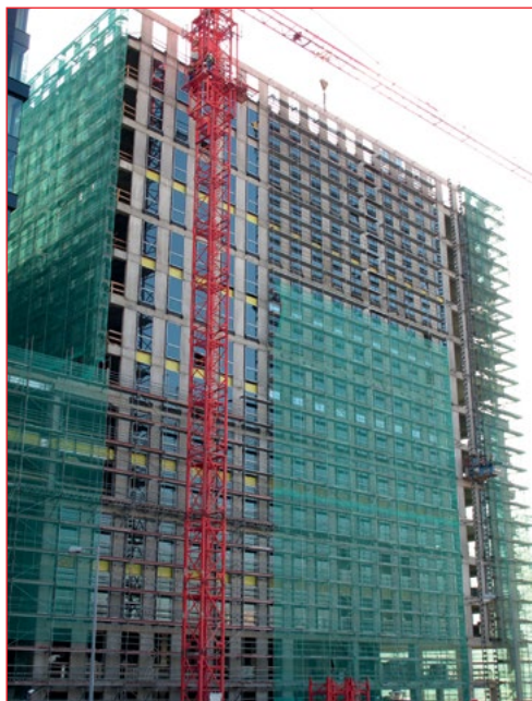
Construction of Quattro Business Park - Cracow
