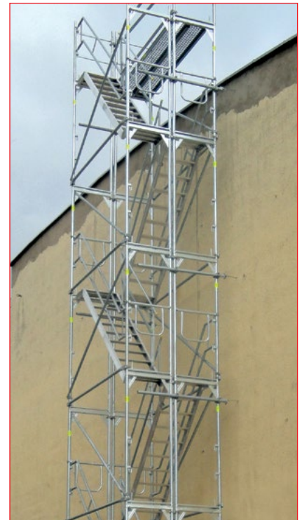
Example - installed double staircase
