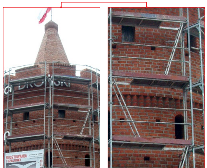
Facade tower's renovation – Szczecin
