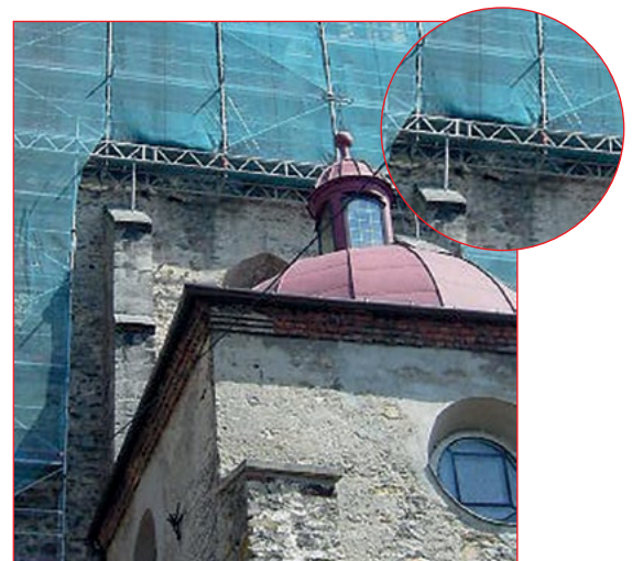
Renovation of the church facade - Szydtowiec
