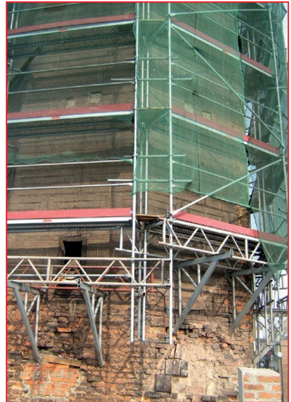
Town Hall in Głubczycze - console 1.5 m
