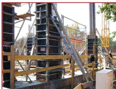
Pole forming – MIDI BOX boards and formwork locks
